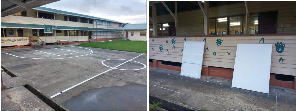
Court marking and backboards being installed at Covent Garden
